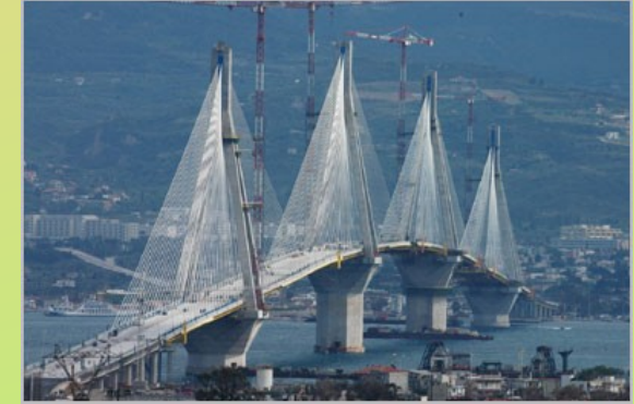
Rion Antirion bridge
